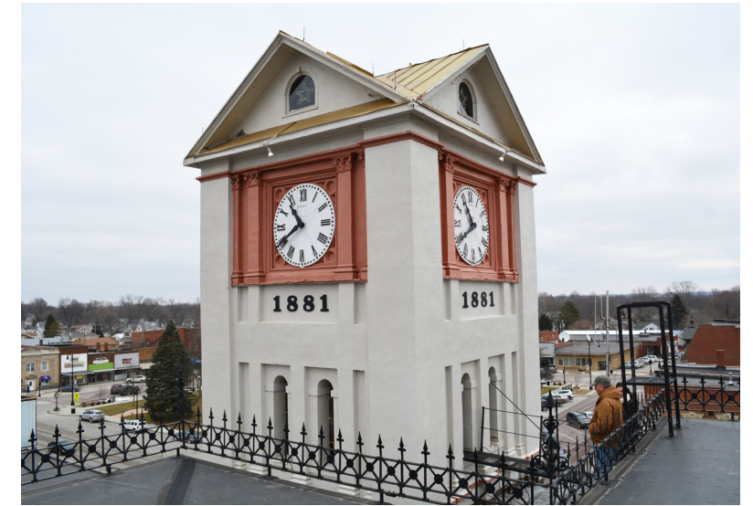
Schuyler County Board President Max McCellon on the courthouse roof with newly restored clocktower and metal cresting.
