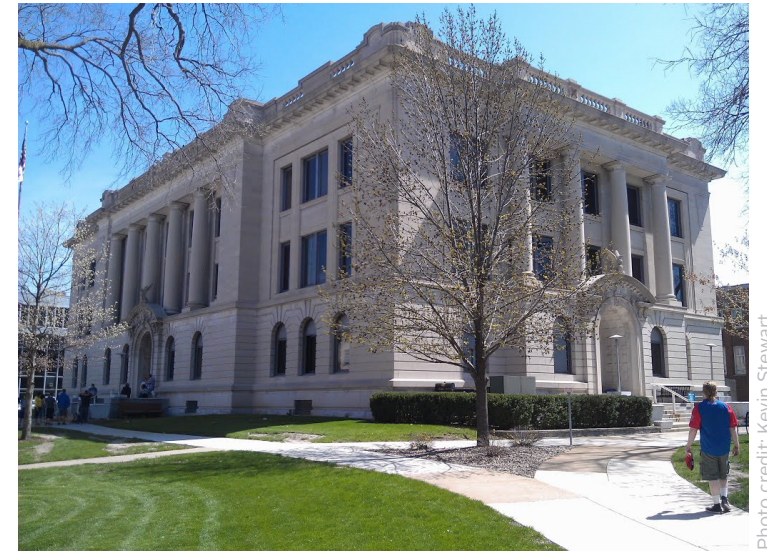
Tazewell County Courthouse prior to lighting project.
