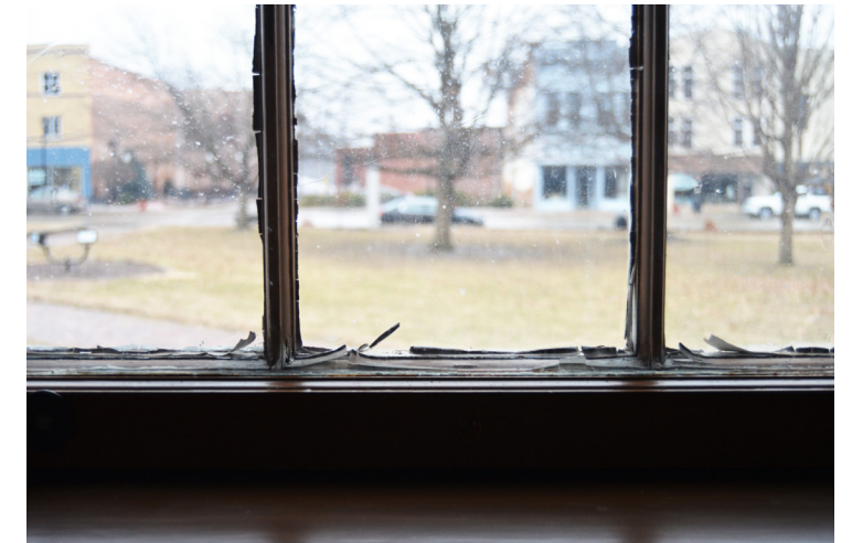
Deteriorating windows on the Vandalia statehouse. Fundraising is underway to restore all the courthouse windows.
