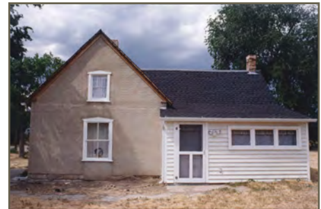
Spring City home after rehabilitation
