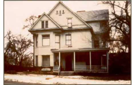
Avenues home before rehabilitation, Salt Lake City
