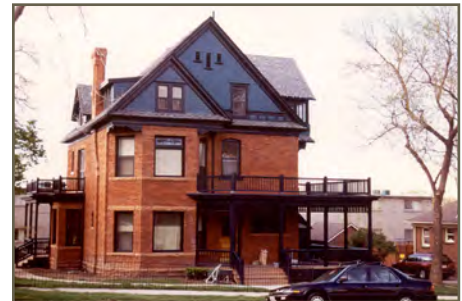
Avenues home after rehabilitation, Salt Lake City
