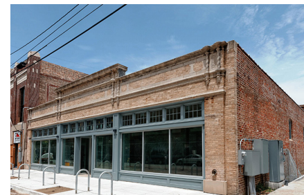
Photo credits: FH Myers Construction
