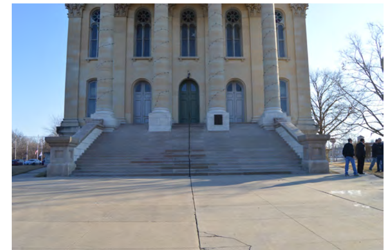
(Top) Macoupin County Circuit Clerk and courthouse historian Mike Mathis shows off the courtroom interior. (Bottom) Macoupin County Board members gather near the newly restored north stairs.
