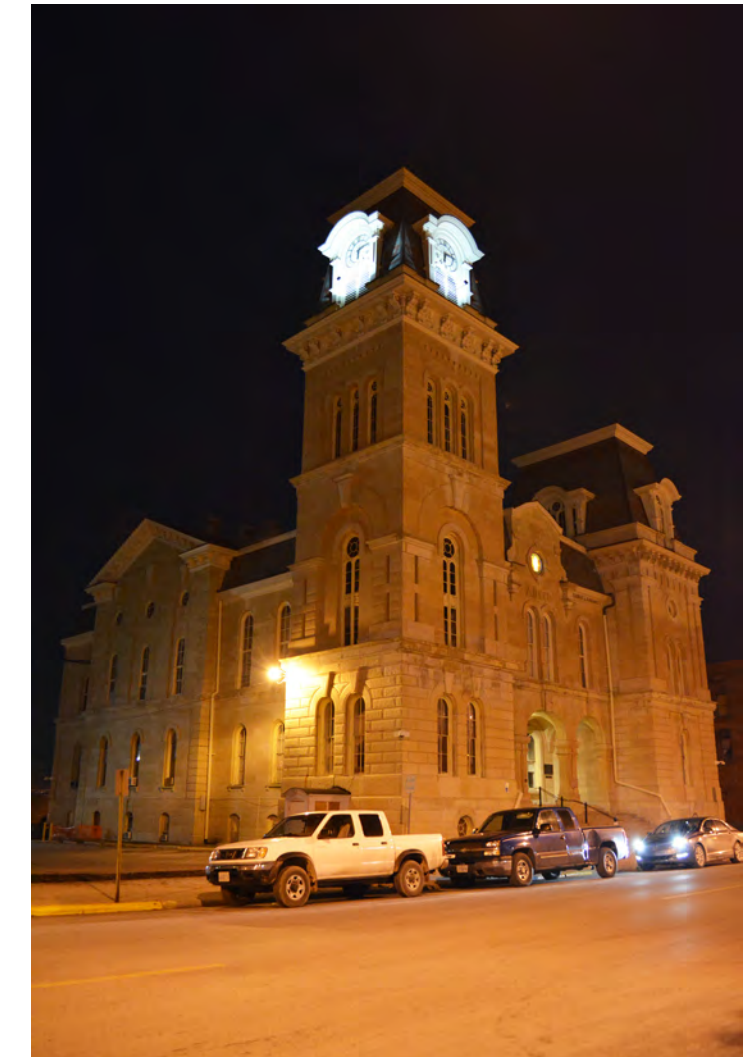
Morgan County Courthouse at night awaiting lighting installation.
