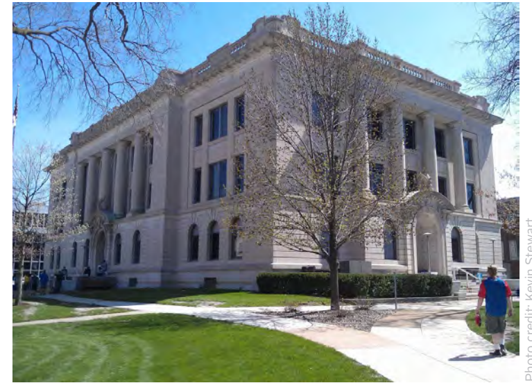
Tazewell County Courthouse prior to lighting project.
