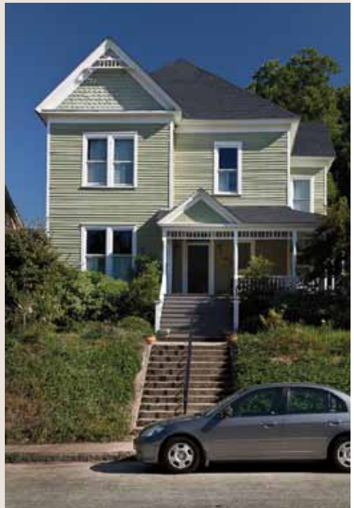
986 Adams Street in Macon before and after rehabilitation. Photo courtesy of Historic Macon Foundation (before) and Georgia Department of Natural Resources (after).
