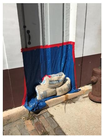
Figure 4.5 Homemade Temporary Flood Wrap Deployed in St. Augustine
