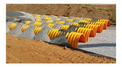
Figure 4.14 Underground Storm Water Detention System (Hydrology Studio 2020)
