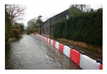
Figure 4.15 Quick Deployable Flood Barrier (Fluvial Innovations 2020)
