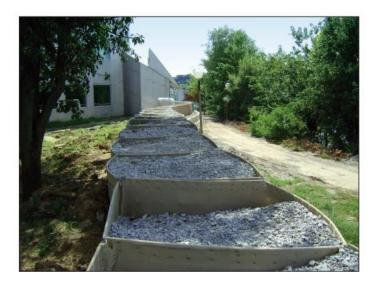
Figure 4.16 Gravel Filled Containers that Form a Flood Barrier (FEMA 2013)
