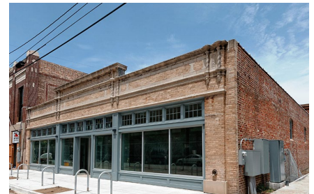
Photo credits: FH Myers Construction
