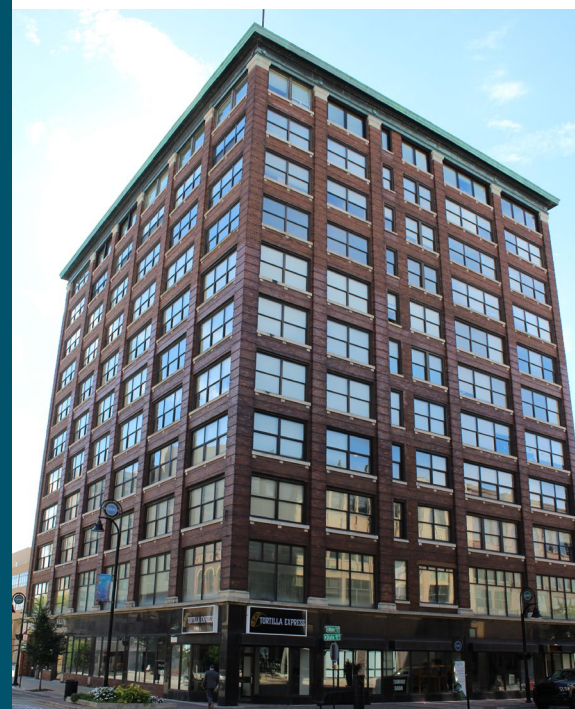
Burnham Lofts (Rockford Trust Building)
